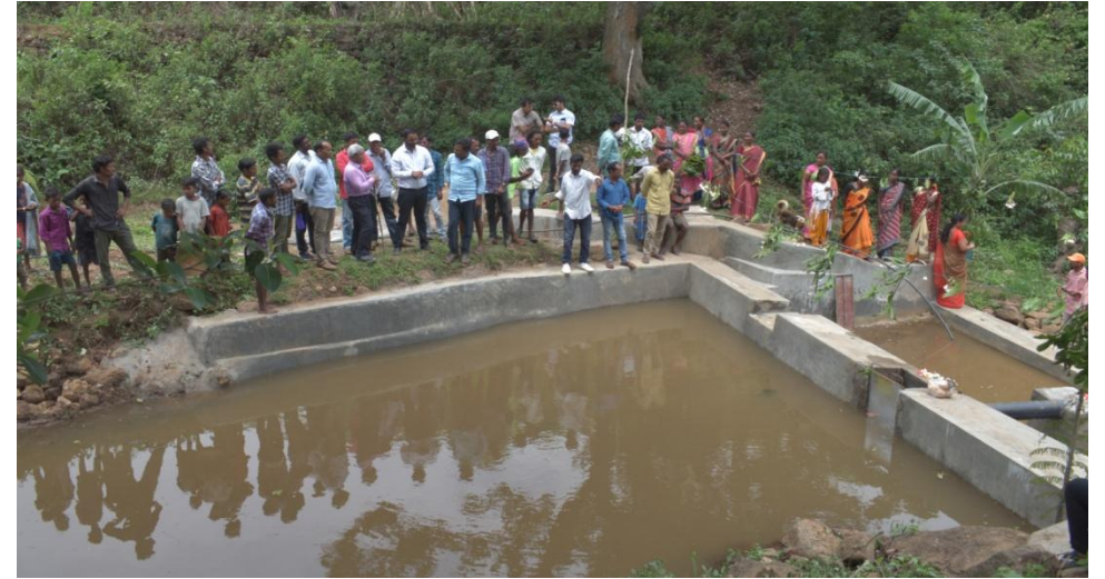
Check dam (Watershed Project) - Minumuluru
